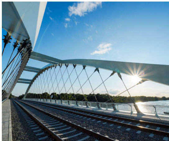
The Oder Bridge and its network arch with a span of 130 metres and 88 carbon hangers Image (left): Volker Emersleben/Deutsche Bahn AG
